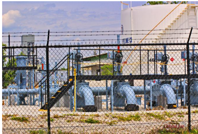
Figure 1 ~ "Colonial Pipeline", Photograph by Orbital Joe
